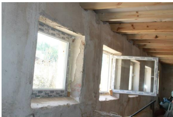
Downstairs – Windows in first section
