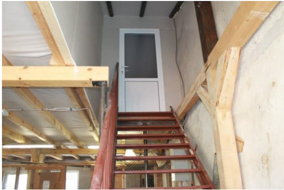
Upstairs – staircase, flooring, windows, door
